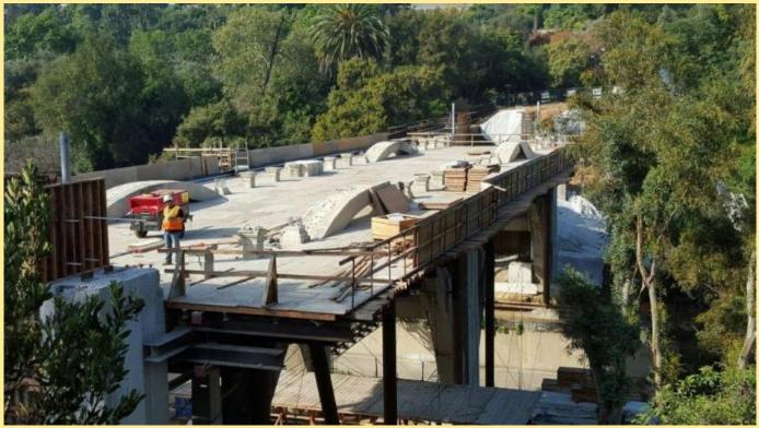
As reported by Pasadena City Engineer Brent Maue, PE: The bridge is on schedule to re-open in December 2016. The bridge demolition work is complete and the contractor has transitioned to the construction of the new sub-structure components. As nearby residents are probably well aware, the contractor has recently been installing driven piles for the support of the west abutment. This process is now complete for the entirety of the project. Current project work includes:
