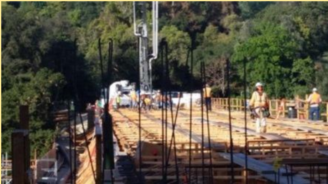
Picture of soffit pour courtesy of the City of Pasadena
